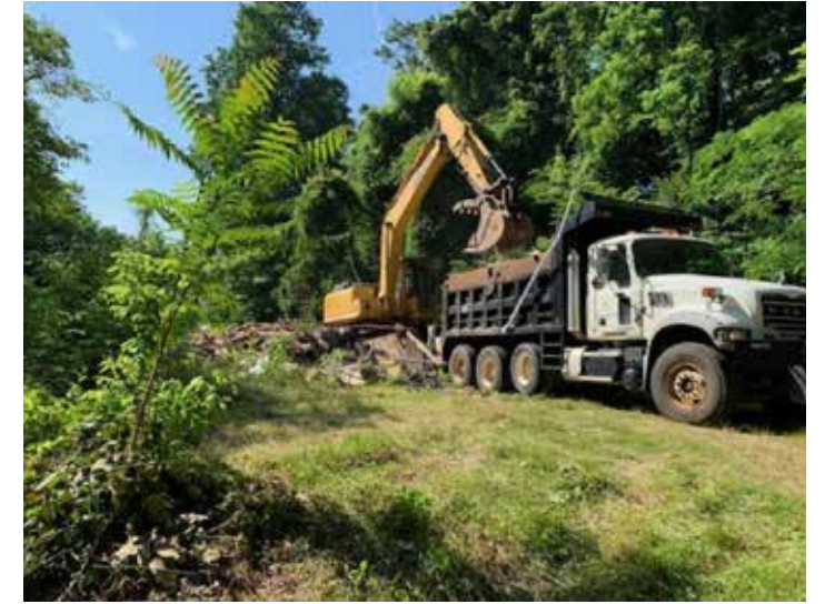
Dunn Street Demolition & Trail build
